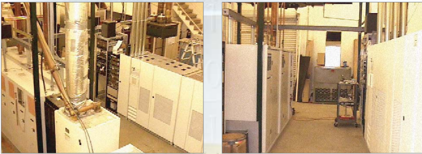
MGE EPS 6000 UPS supporting an IOT transmitter. This site has experienced numerous crowbars with the UPSs managing the fault without incident.
